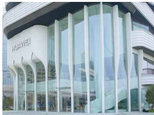
Huawei Taikoo Li Flagship Store · China
